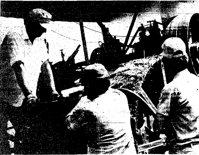
PITCHING BUNDLES is hot work for Russell Johnson, above. Power for the threshing is transmitted from the steam engine by a 50-foot belt. Below, Carl Johnson chats with Don Pederson and Tim Reese, Omaha, during a break to take on water for the steam engine which provided power for Saturday's threshing show.
